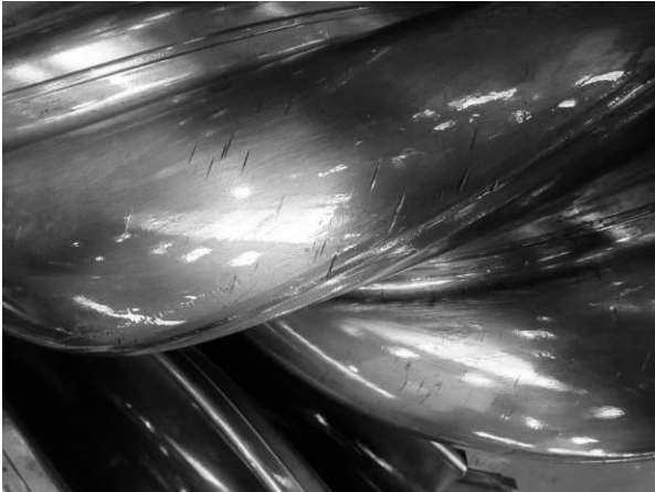
Fig. 5: Marks (male rotor) due to dirt
